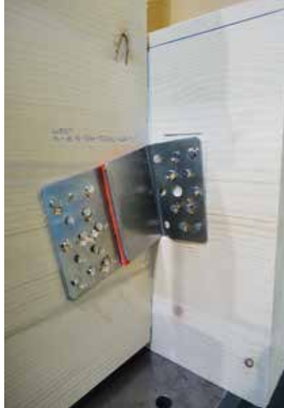
^ Figure 3: Typical, predominantly ductile failure of the Sonus sound insulation angle
